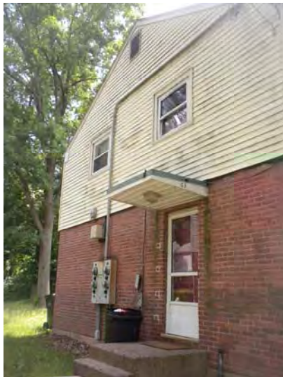
Typical unit entryway with original door, older aluminum storm door, and canopy
