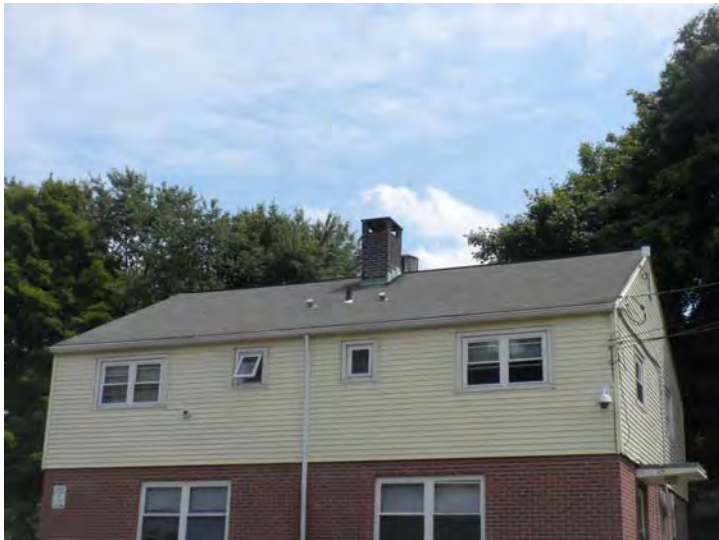
Typical asphalt shingle roofing
