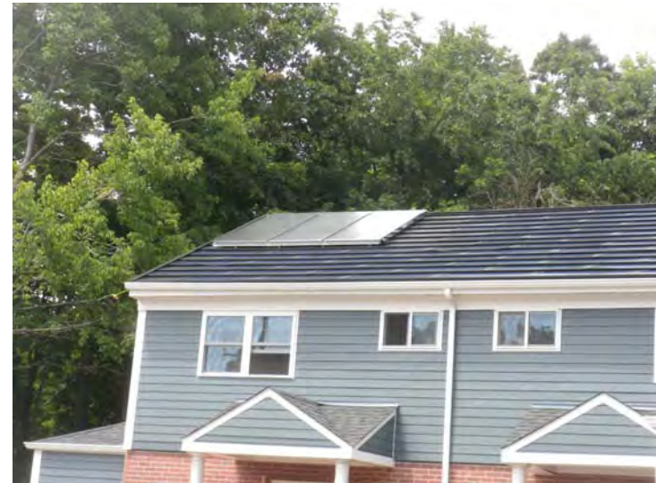
View of the solar photovoltaic shingles and solar thermal panels at the rehabbed building
